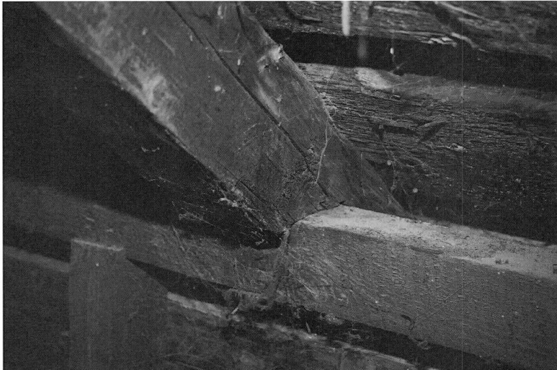
Photo 11 of 13: Attic, rafter foot/plate connection. 1/14/2022
