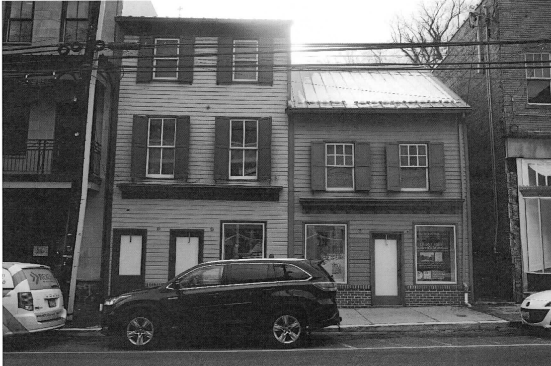
Photo 1 of 13: North elevation, 8109 & 8113 Main Street. 1/14/2022
