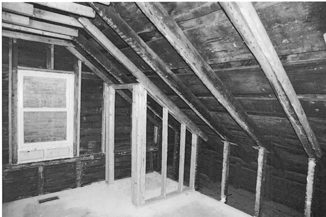
Photo 9 of 13: Attic, view northwest. 1/14/2022
