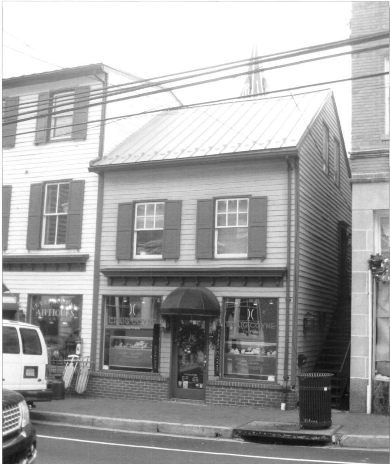
HO-359 Caplan's Frame Shop (Crosscurrents) 8113 Main Street (MD 144) Photo by Jennifer K. Cosham, 12/5/2012 North elevation
