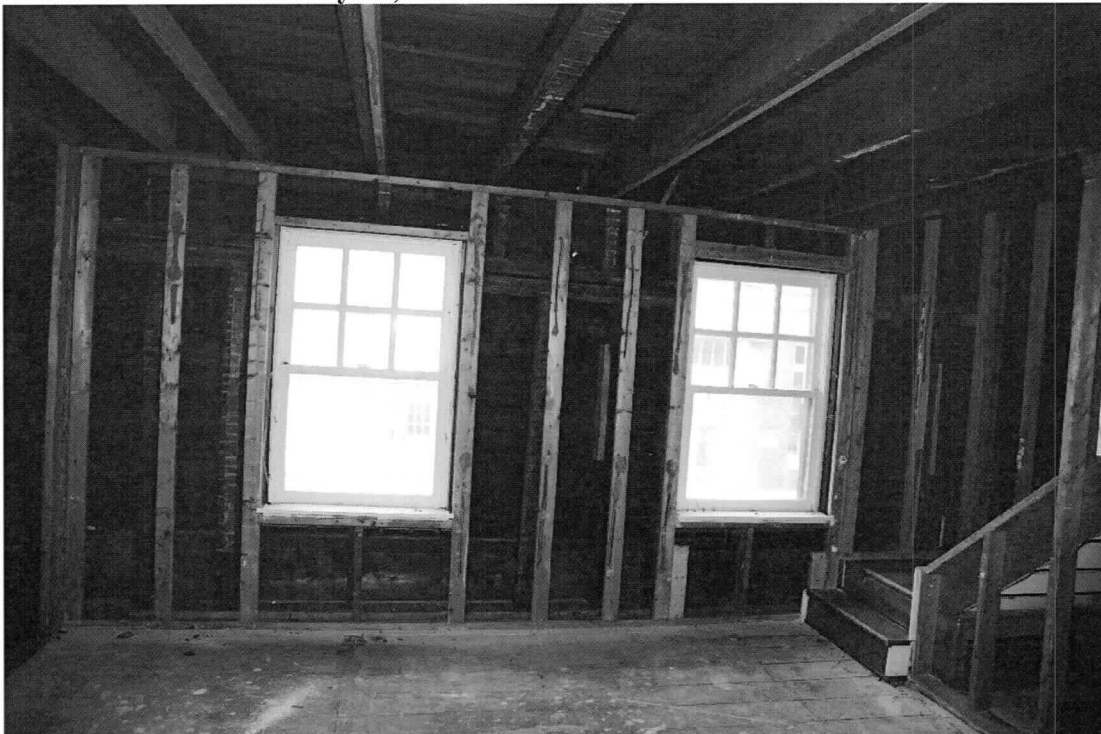
Photo 6 of 13: Second story north wall. 1/14/2022
