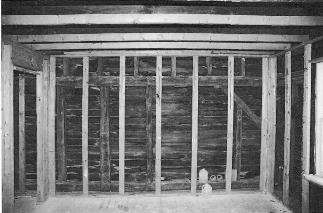
Photo 7 of 13: Second story west wall. 1/14/2022
